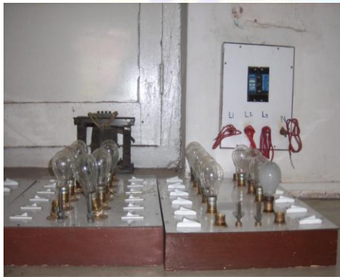
Figure 2: 3-Phase Supply and Lamp- Boards
